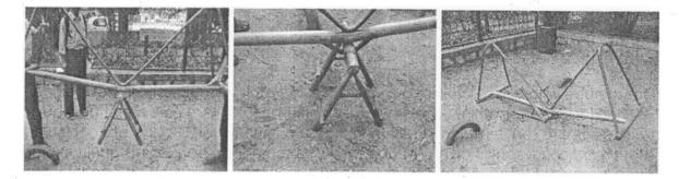
The play equipment (FRP portion) has also been worn out within a year leading to a unsafe situation. The 4 seater swing has only two swings working! The seat is anchored by only 3 hooks. See photos
