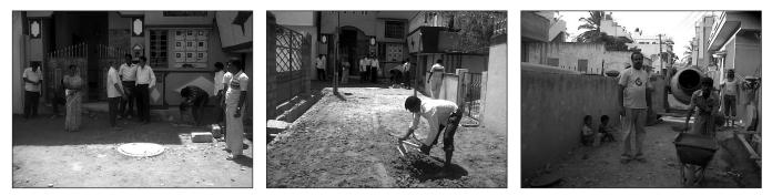
In 3rd Main, women volunteers of the association monitored the work. They also identified the low quality work, such as the reduced thickness of the asphalting work done. As per the estimate, the contractor was supposed to put nine inches of asphalt; instead, he was putting only four inches. Again, women volunteers informed key leaders of the association and the AEE. The AEE inspected the work and promised the members that he would instruct the contractor to set right the work.
